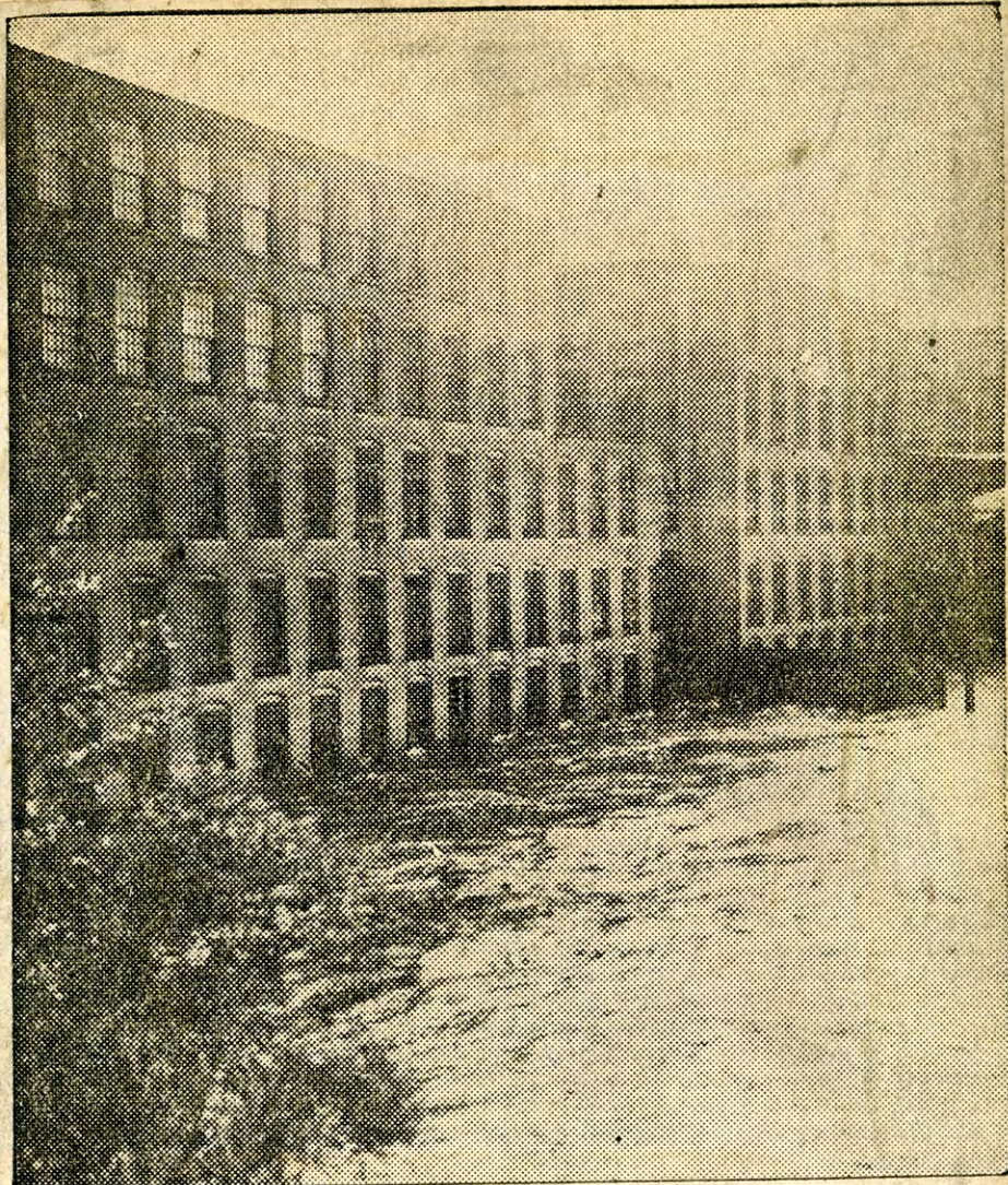
FALLS WESTINGHOUSE PLANT MAROONED: CHICOPEE Falls Westinghouse was walled by water, which at this point was 30 inches deep inside the buildings.
