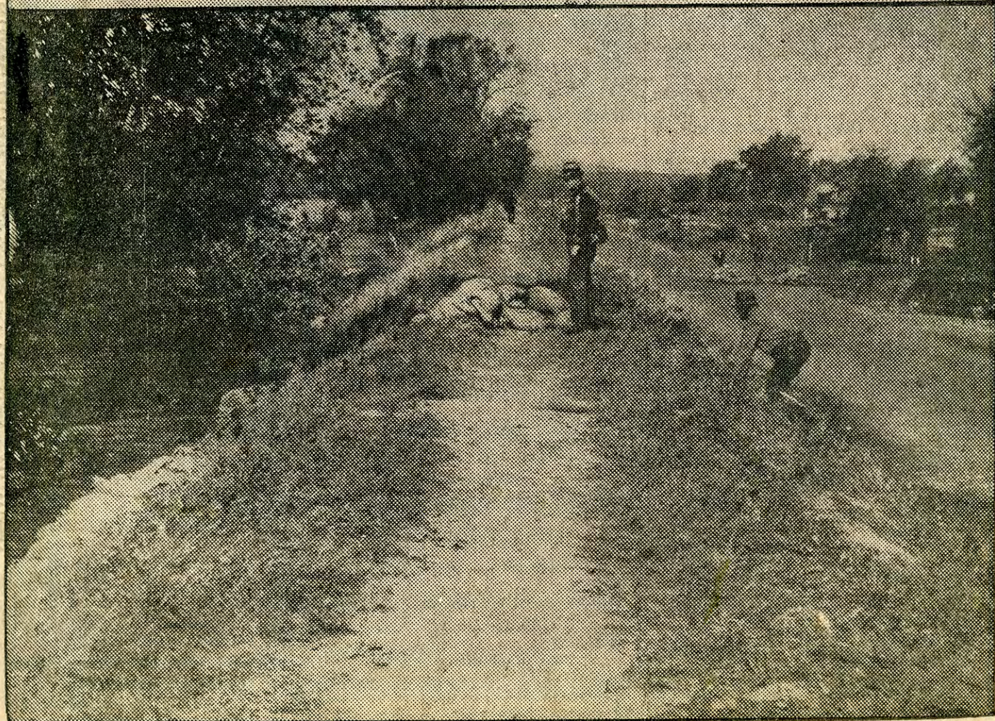
Upper, dike opposite Washburn-street pumping station; lower, placing sandbags on the dike.
