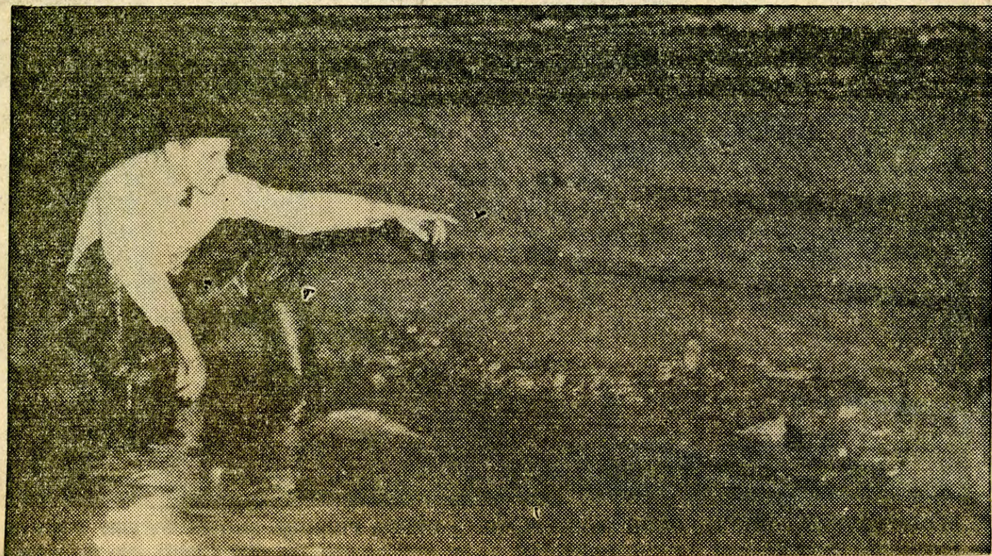
WASHOUT ON BOSTON ROAD NEAR NO. WILBRAHAM.
