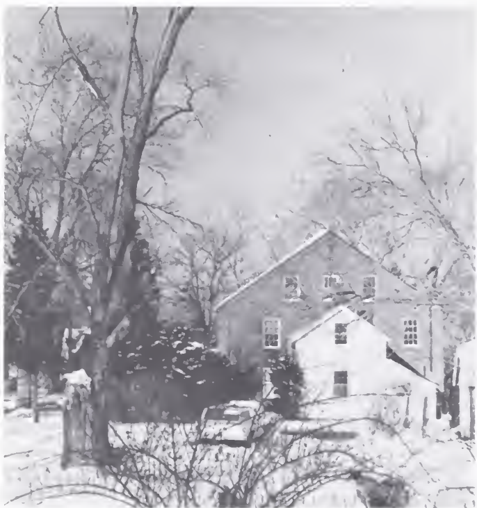
"The white wooden structure was the oldest of the two buildings."
