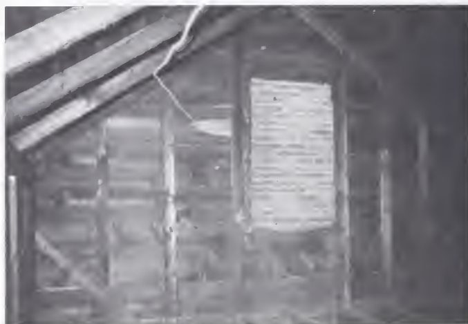
"A bricked over window at the end of the wooden house wall, was found to date back earlier than the house itself."
