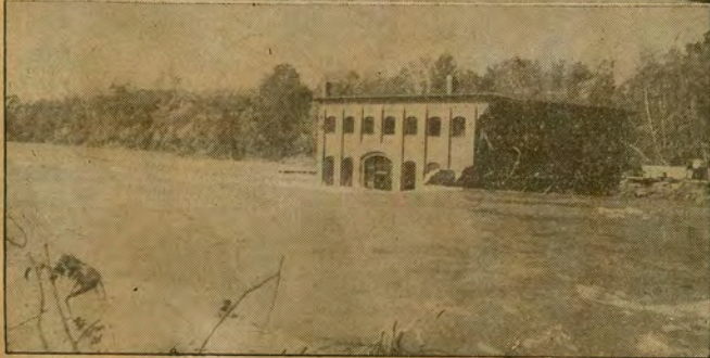
BIRCHAM BEND POWER STATION BEFORE AND AFTER. THESE PICTURES TAKEN FROM the same point in Bircham Bend road showed what the flood in Chicopee river did to the power plant of the Quinnetuck Power company. The main entrance of the plant can be seen through the shade trees before the river cut a new course, washing away with it the home occupied by a company engineer, Theodore Parent. Mrs Parent had just returned from the hospital and had to be returned to the hospital when the floodwaters swept around the house. Several men were required to carry Mrs Parent on a stretcher above their heads through the water, to get back to high ground.
