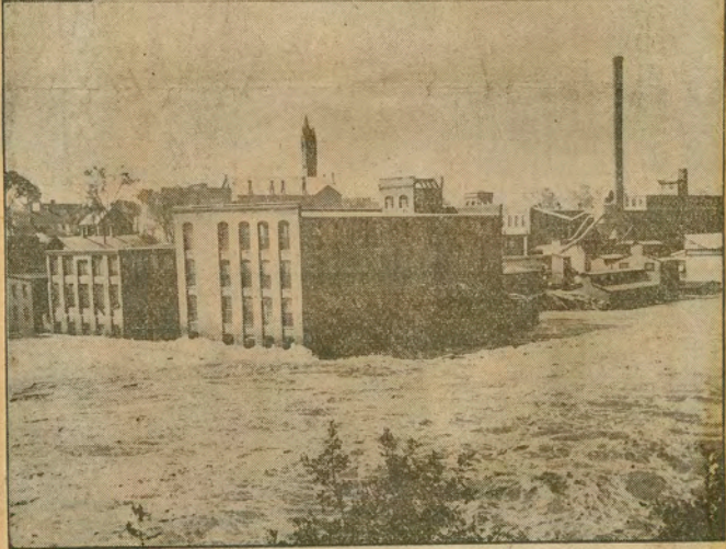
DAMAGE DONE BY FLOOD AT CHICOPEE FALLS. UPPER, RUINS OF CHICOPEE FALLS bridge; center, Westinghouse property under water; lower, Spalding Mfg. Co.
